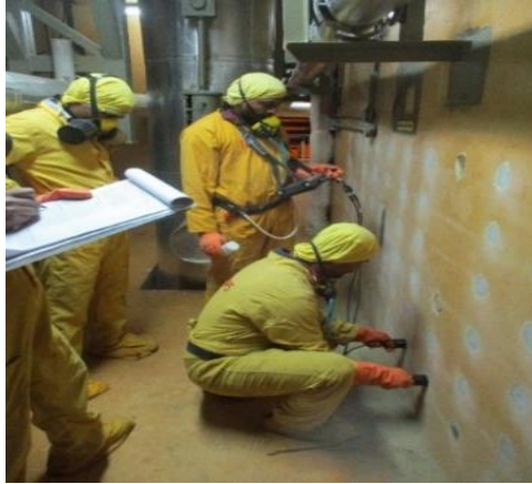
NDT Services provided to a Public Sector Enterprise under the control of Department of Atomic Energy for structural Health Assessment of unit 3 and 4 of a Power Plant. The scope included comprehensive quality check of civil concrete structures.
