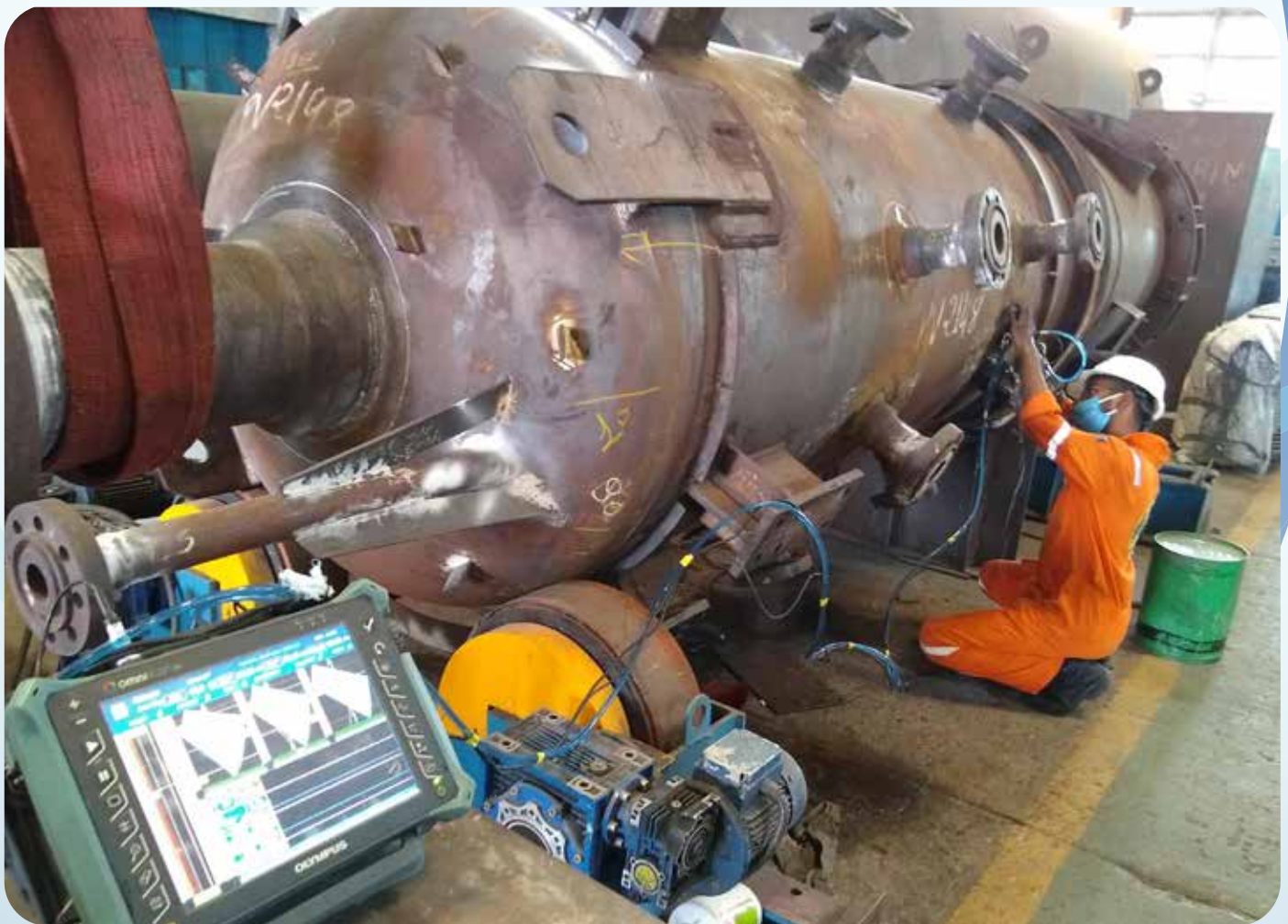
Phased Array Ultrasonic Testing (PAUT) on a fabricated assembly of a pressure vessel
