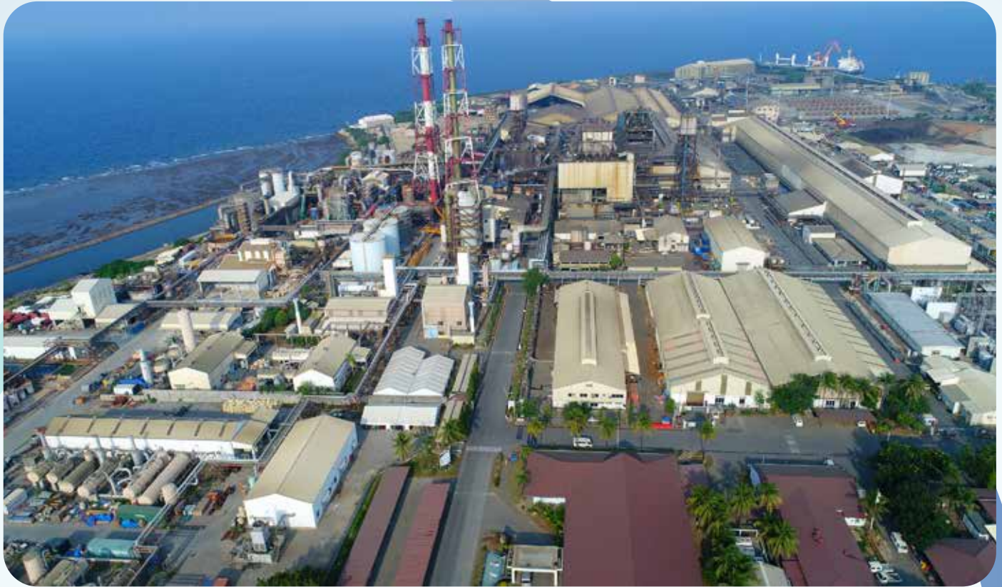
Structural Assessment of All Concrete & Steel structures - PASAR
