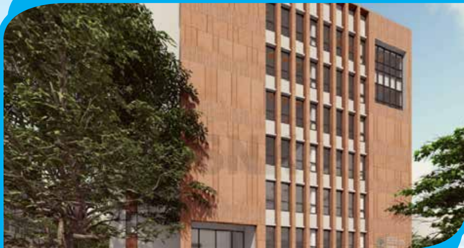
Construction Supervision at IIT Bombay New Annexe to HSSA Building.
