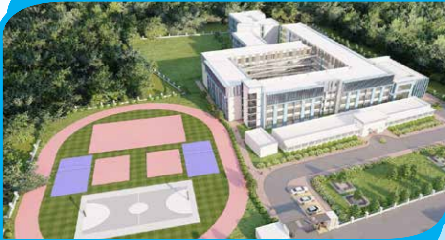
Construction of Primary School Building under CM RISE Project - Madhya Pradesh Building Development Corporation Bhopal.
